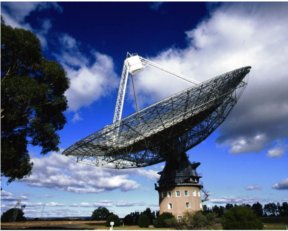
Single-dish telescope: \text{cost} \propto A^{1.35}
